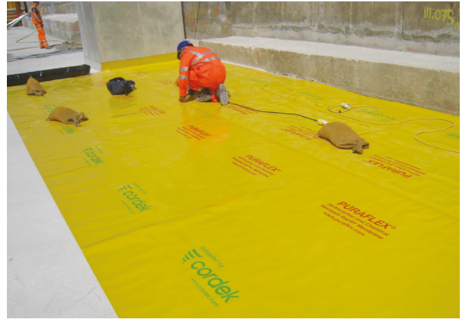
Membrane being installed
