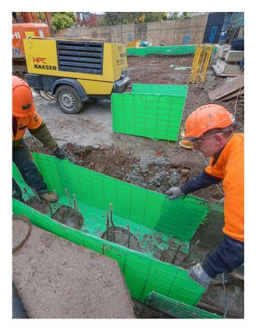
The project at Lonsdale Road consisted of demolishing the existing three storey building and replacing it with a terrace of three residential dwellings. Cordek were asked to supply a permanent formwork system for the construction of the reinforced concrete foundations.
