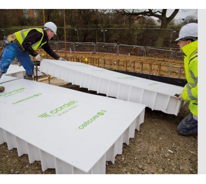
Cellcore HX is Cordek's fourth generation collapsible void former and has been designed to protect foundations from the effects of ground heave.
