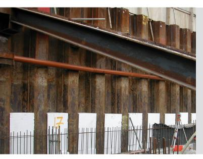
Sheet Pile Infills are designed as a quick, economical and lightweight solution to infilling the open pans in an exposed sheet pile wall. Manufactured to order from Filcor EPS, they are available in a range of profiles and densities to suit customer requirements.
