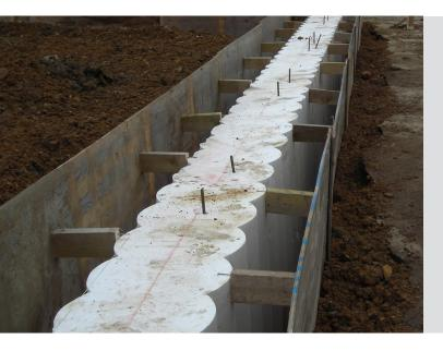
Sacrificial Guide Wall Formers are used to accurately form an insitu concrete guide wall which is critical in the positioning and alignment of piles in a contiguous or secant piled wall.
