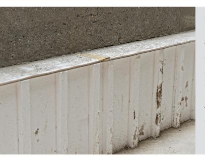
The range of products are available in a variety of depths and grades to suit the most commonly encountered combinations of soil heave potential and concrete depths that exceed the capacity of the standard Cellcore HX range. If a suitable product for your requirements is not listed within this data sheet then please contact our sales support desk for further assistance.
