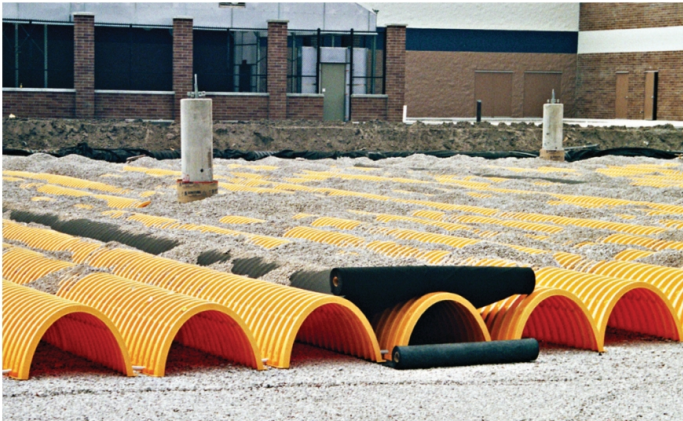
The ADS StormTech system has a built-in water quality treatment device
