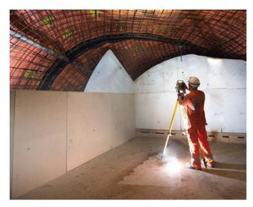
The formwork concept was installed in stages to suit the preferred concrete pour sequence required for this complex structure the fibreglass coating was applied and the plywood backing bonded into position. The formers were manufactured and delivered in three stages over an eight-week period to suit the contractor's programme.
