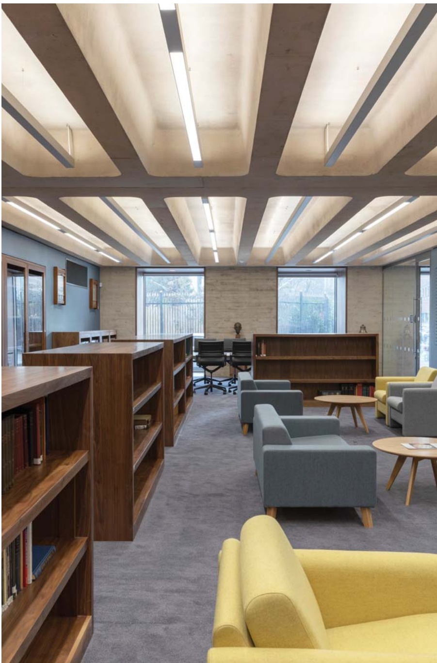
LEFT: Exposed concrete surface finish with one-way spanning ribs at Royal College of Pathologists.
