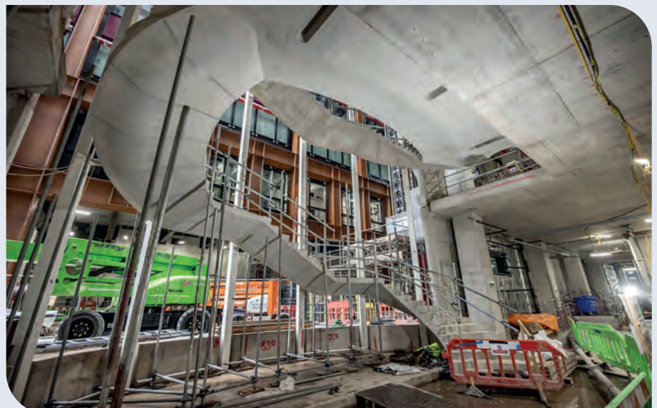
ABOVE: Another view of the helical stair for Salisbury Square Development.
