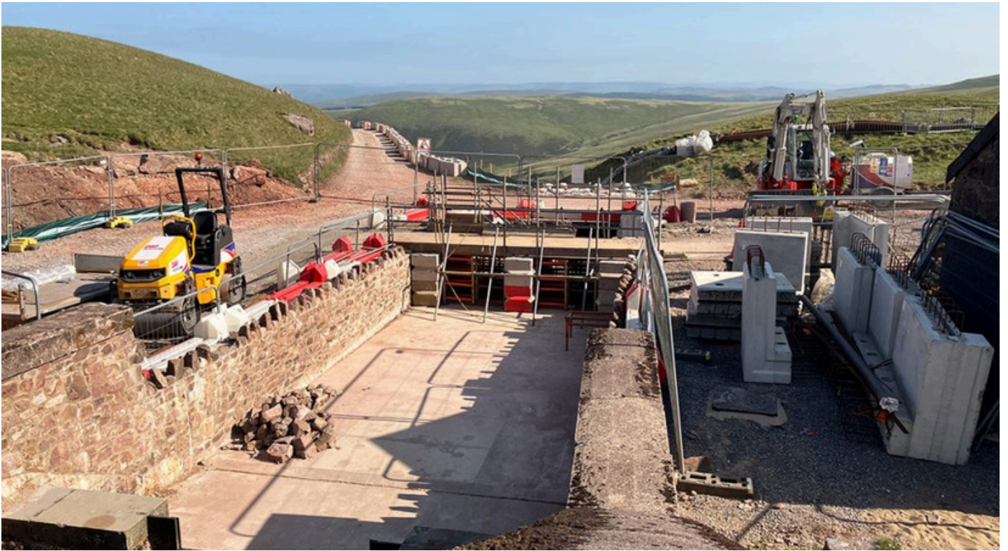
Spillway construction and lining – Courtesy of Morgan Sindall
