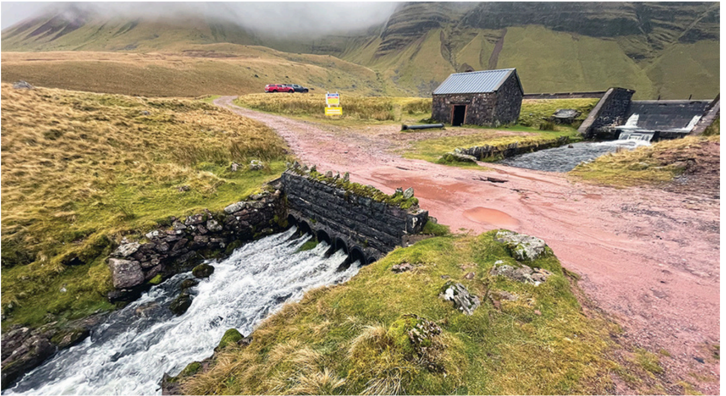
Spillway prior to works – Courtesy of Arup
