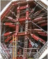
at an angle. This required the Filcor 70 EPS segments to be tapered so that the RMD Kwikform frame could remain a consistent profile throughout. The RMD Slimshor frame was set perpendicular to the main wall with the incoming tunnel at an angle, requiring the tunnel lining the inner face and curved to form the surface of the concrete ring externally.
