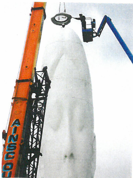
Figure 6: Positioning of final precast unit.
