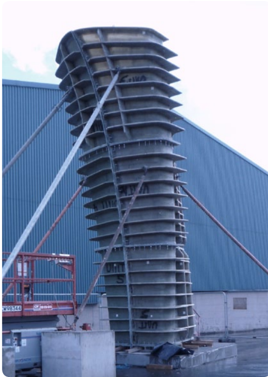
Figure 8: Dive towers under construction showing 5m board in the foreground, 10m board behind and the restricted crange and access.
