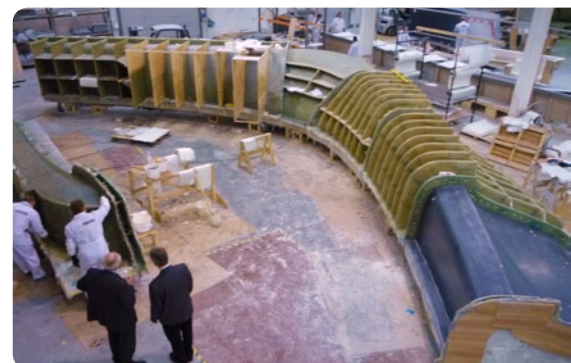
Figure 6: Formwork units in various stages of construction.
